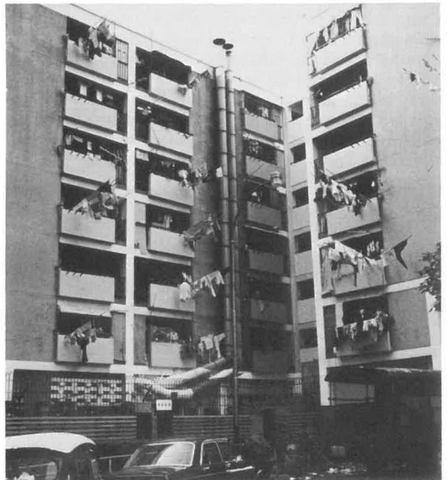
Restaurant chimney in the midst of public housing.
